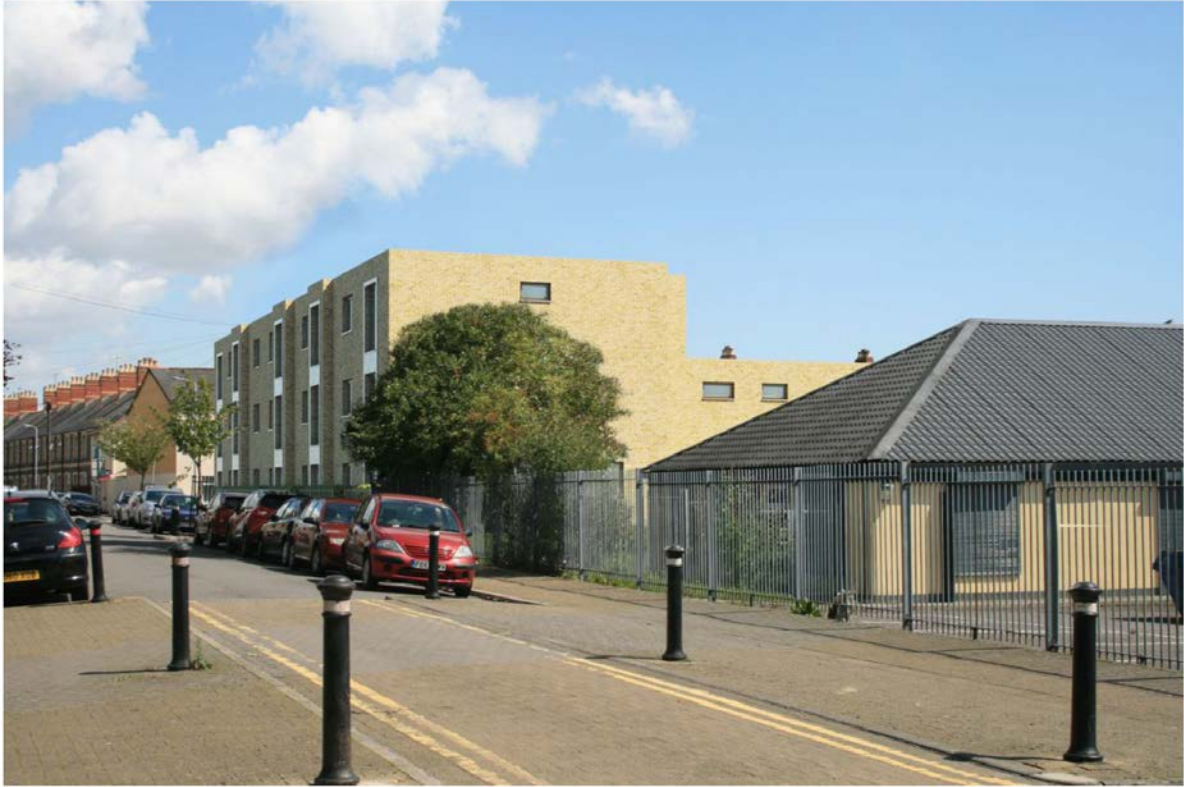
View looking east from Sun Street
