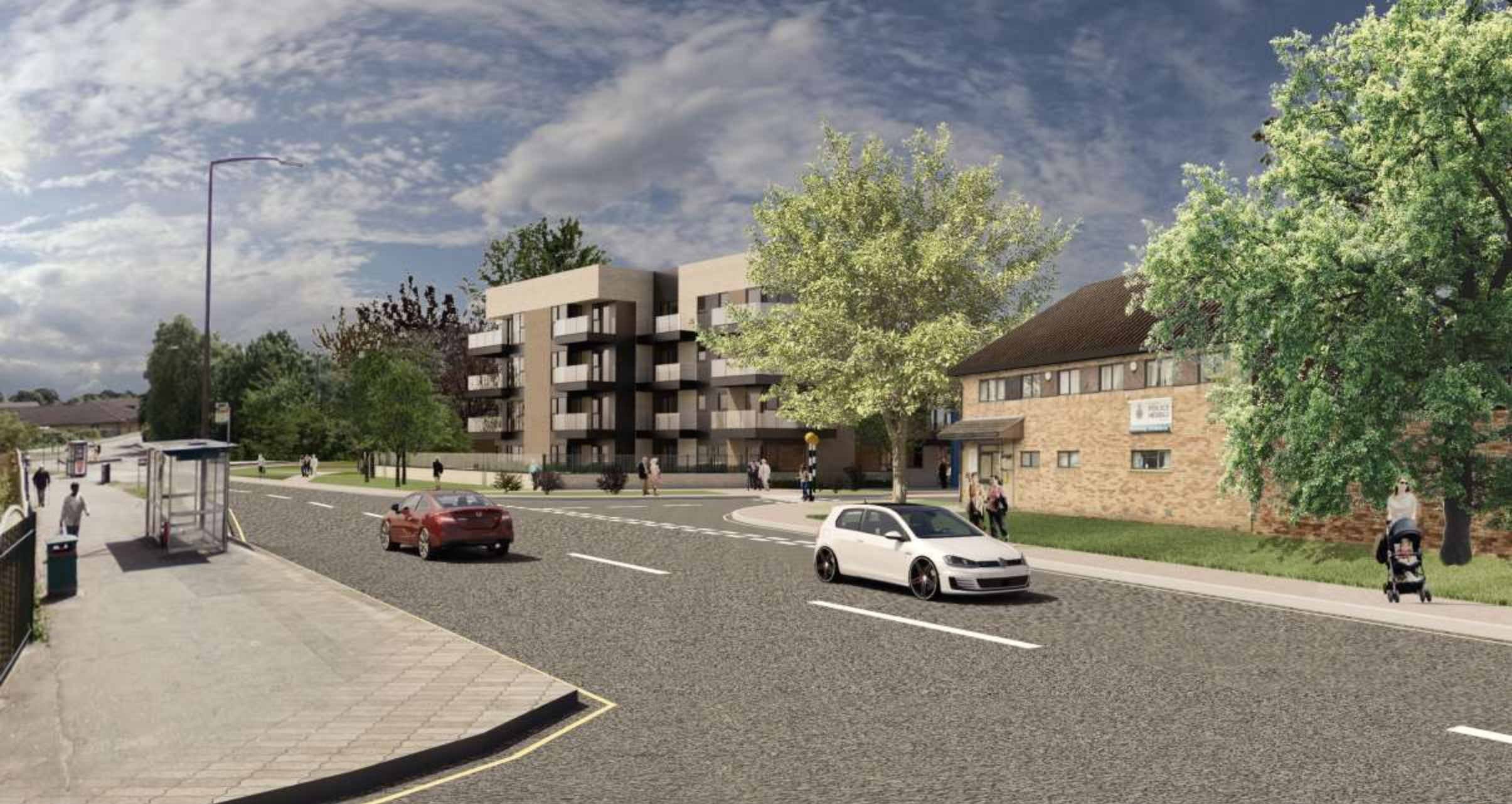
View from Junction of St Arvans Crescent - Crickhowell Road
